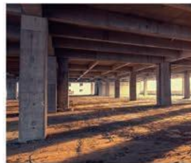
Finish Construction Survey
